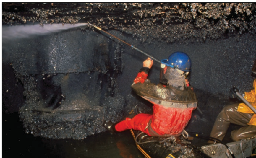
Figure C.19 Masked workers use a water jet to clear zebra mussels clogging the walls of the pump room of Detroit Edison's power station in Michigan, USA. Not only do zebra mussels encrust water pipes and pump rooms, but they also excrete a corrosive substance.
